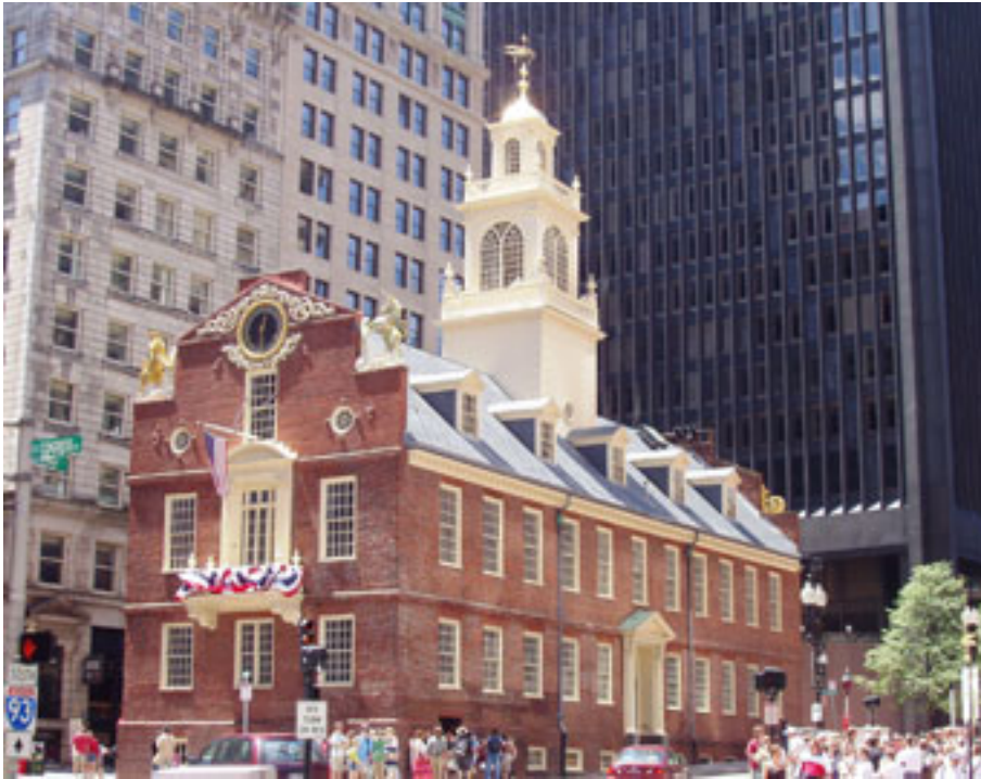
Figure 26 An old house among newer buildings
